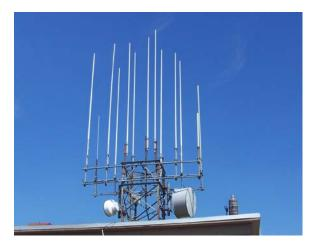
level. In our example, if we double the distance between the antennas, the signal levels will drop by 6 dB and any intermodulation products produced by those fundamental signals will drop up to 18 dB.
